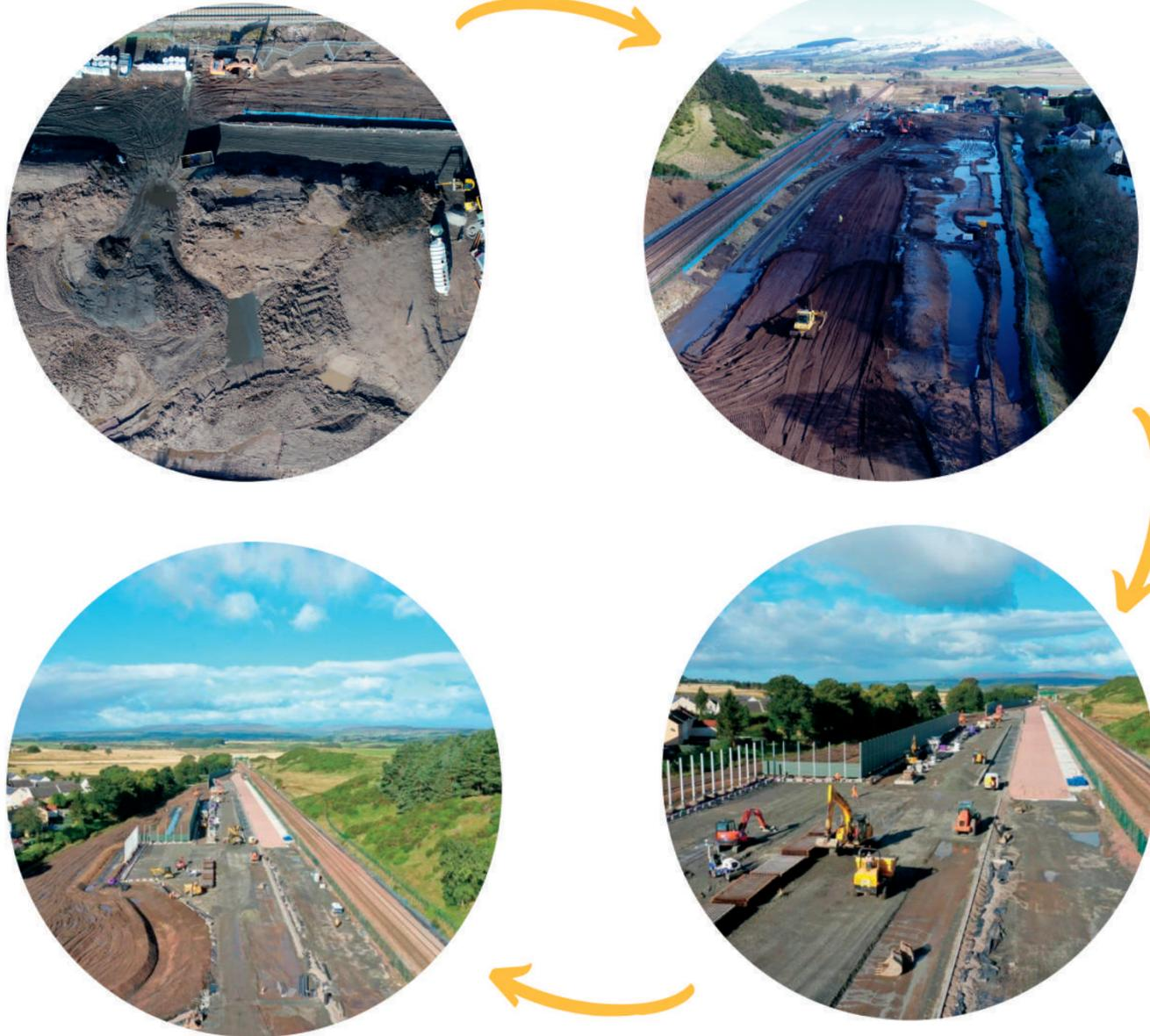
Rather than disposing of the 25,000m<sup>3</sup> unsuitable soil in landfill, ATG Group proposed to stabilise the soil.
